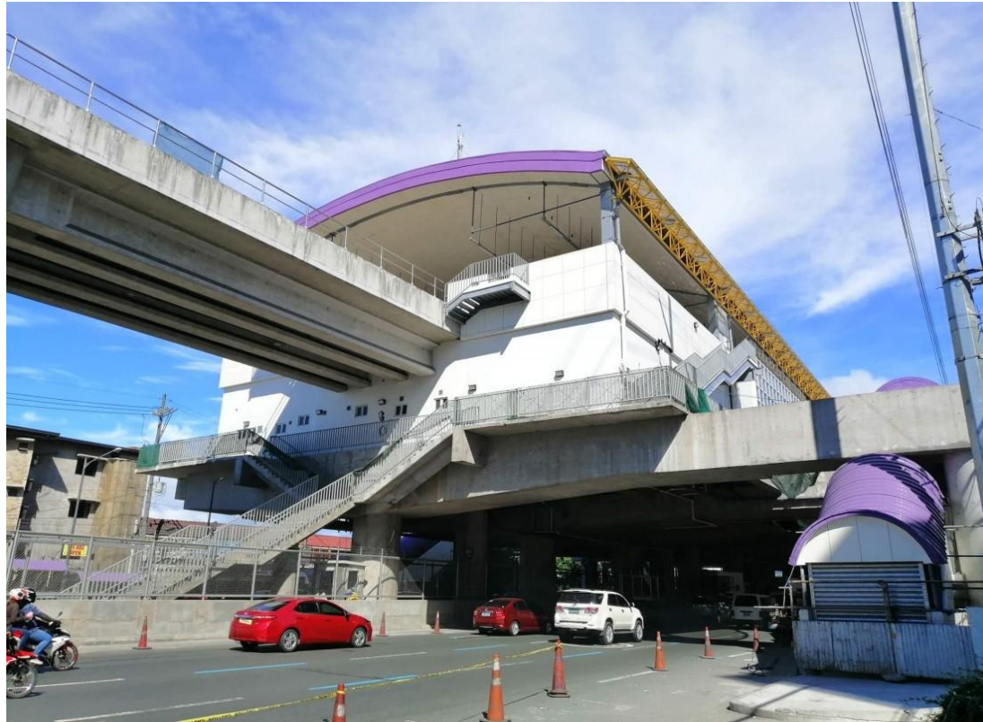
Marikina Station (Street Level)
