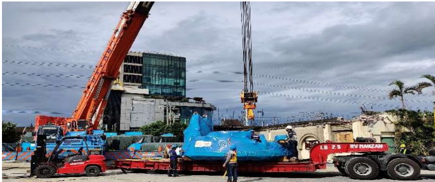
TBM Stockyard at Tandang Sora
